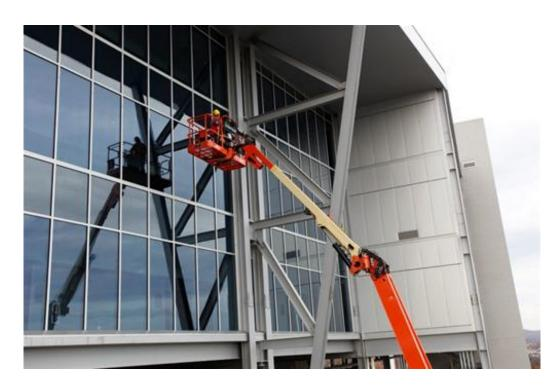
Telescopic Upper Jib – extends from 4.65m to 7.62m with 120 degrees (+75 / -45 degrees) vertical range of motion.
