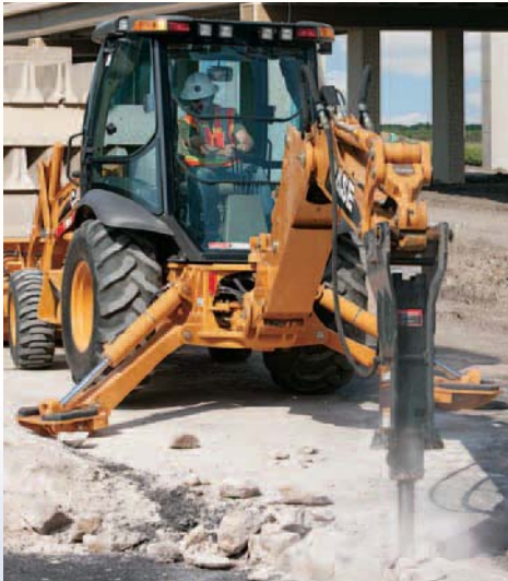
Optimized hose routing for demolition work
